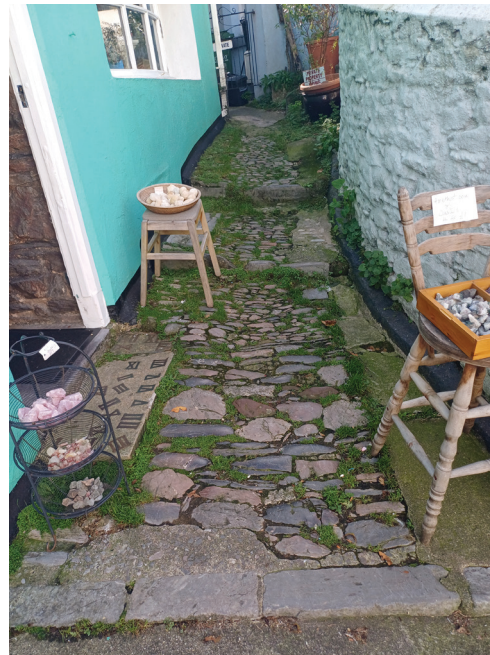
Historic surface finish to a private lane off The Strand.
