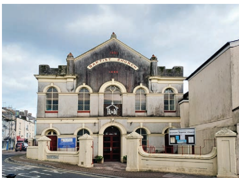
Baptist Chapel on Market Street, begun 1801.
