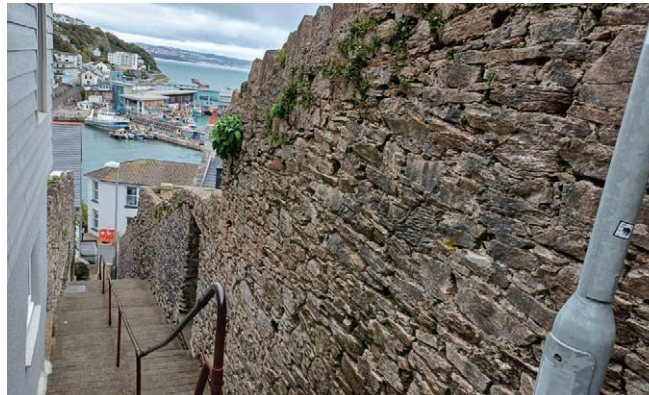
Exposed rubble stone wall at Queens Steps.
