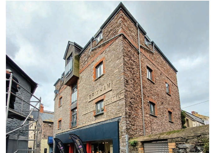
A former industrial structure off Pump Street.
