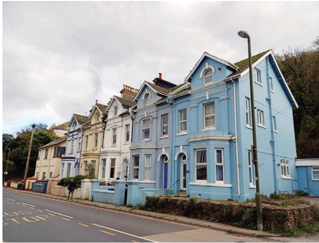
View 17: A later 19th-century terrace on New Road.
