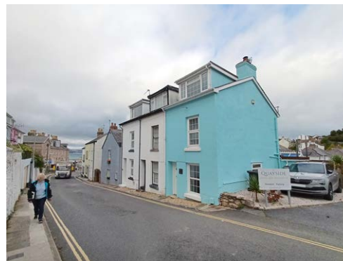
An early 19th-century terrace on Ranscombe Road. Note the uniformity of the fenestration across all three houses.
