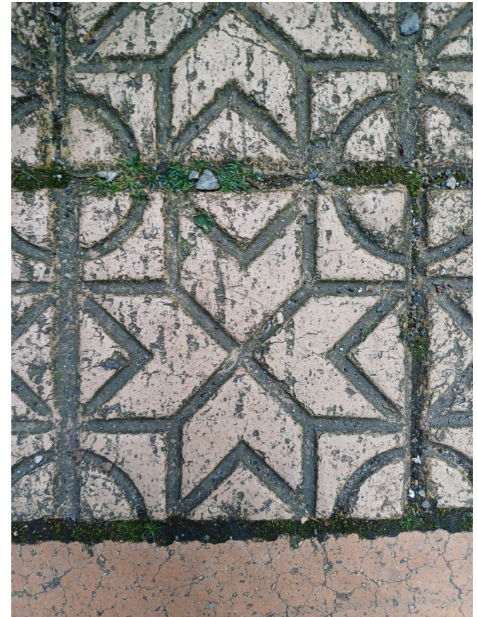
Detail of the late 19th-century decorative pavers found throughout the conservation area.
