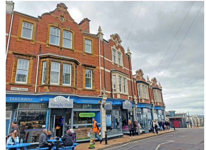
Edwardian commercial structures on the north side of Fore Street/The Strand.
