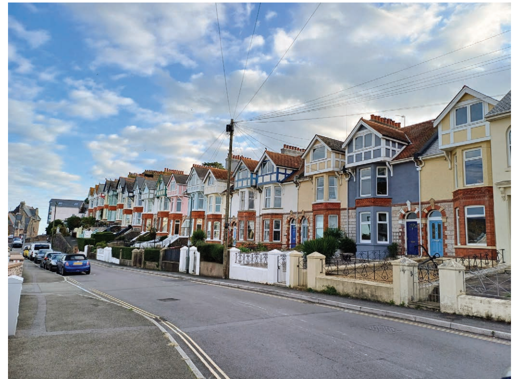
Edwardian terraces on Berry Head Road. The use of mock close-studding to the gables and hung tiles are typical of early 20th-century domestic architecture.
