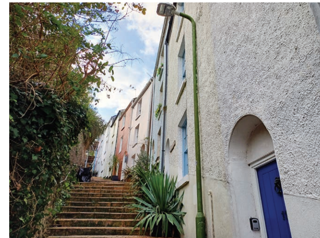
Early 19th-century terrace at Temperance Place.
