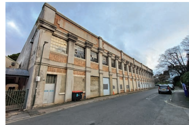
The east elevation of the former interwar coach depot, between Torwood Street and Torwood Gardens Road.
