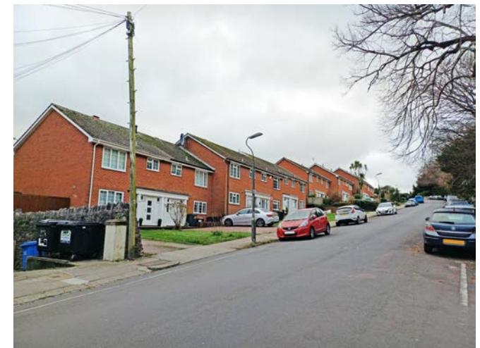
Modern terraced development at the top of Braddons Hill Road East.
