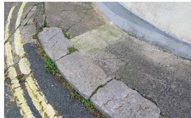
Local limestone and slate can be found in kerbstones across the conservation area.
