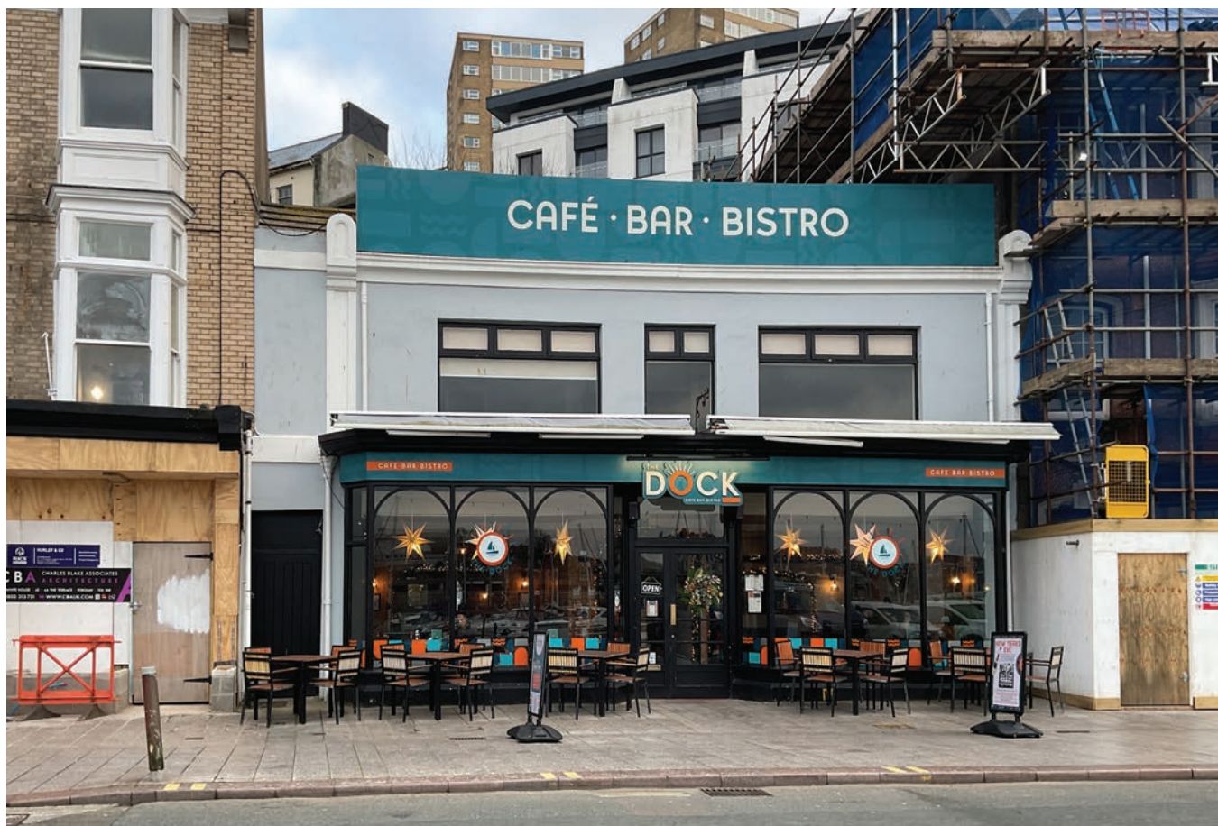
A traditionally styled shopfront on Victoria Parade, which makes a positive contribution to the streetscape. Reducing the size of the large fascia at the top of the building could further improve its historic character.
