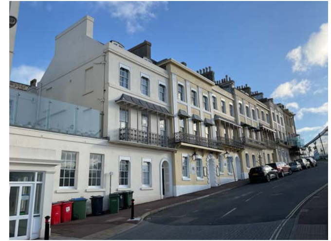
View 29: Looking up Beacon Hill towards the Georgian terrace.
