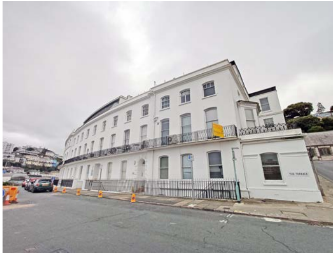
View 28: The Terrace of 1811, viewed from the eastern end.
