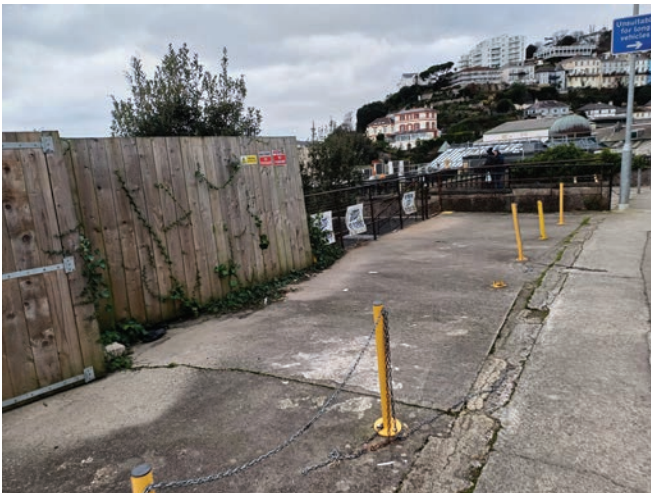
A range of detracting modern boundary treatments to an area of hard standing opposite Higher Terrace, on The Terrace.
