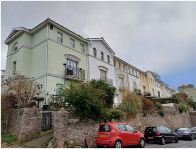
View 27: Mid 19th-century terraces on Montpellier Road.
