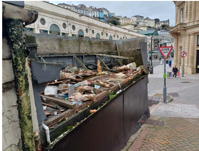
Refuse accruing behind single-storey shops on Fleet Street, at the junction with The Terrace. On the left is a badly deteriorating downpipe.
