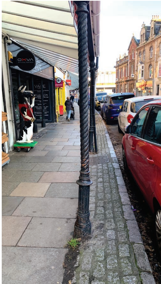
The cast iron columns of the former department store on Palace Avenue.
