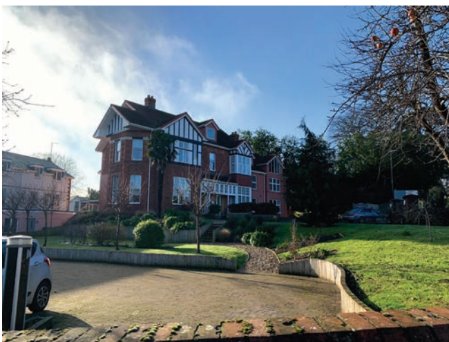
A substantial house on the corner of Totnes Road and Midvale Road with mock timber close studding to the gables and a distinctive timber porch, now converted into assisted living accommodation.
