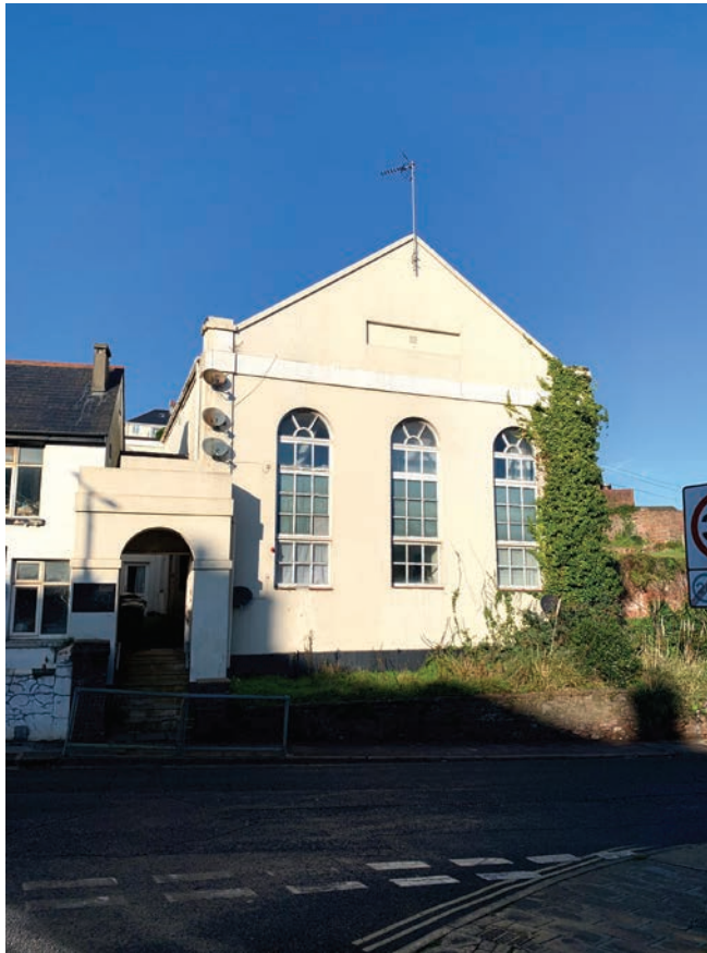
The former Baptist chapel on Colley End Road in a simple neo-classical style.
