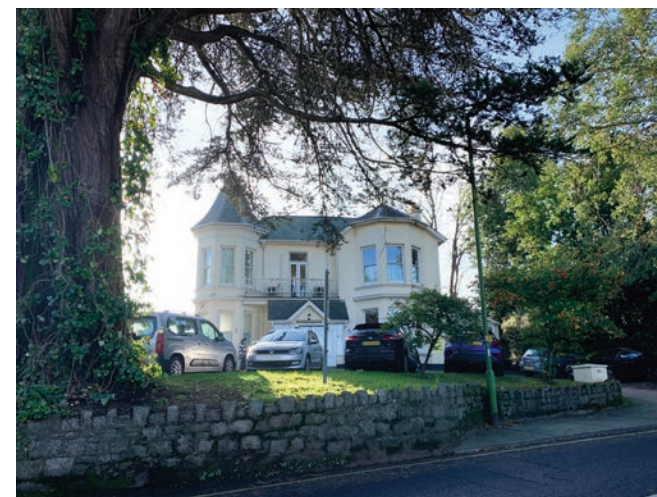
A mid-19th-century house on Totnes Road with corner turret and wrought iron balcony.
