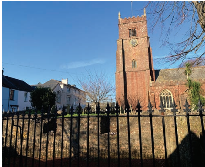
View 18: Church of St John the Baptist as seen from Church Path, looking north.
