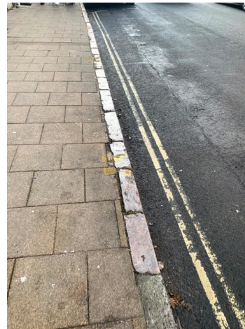
Surviving historic kerbstones on Palace Avenue, with replacement modern slabs to the pavement and tarmacked road.
