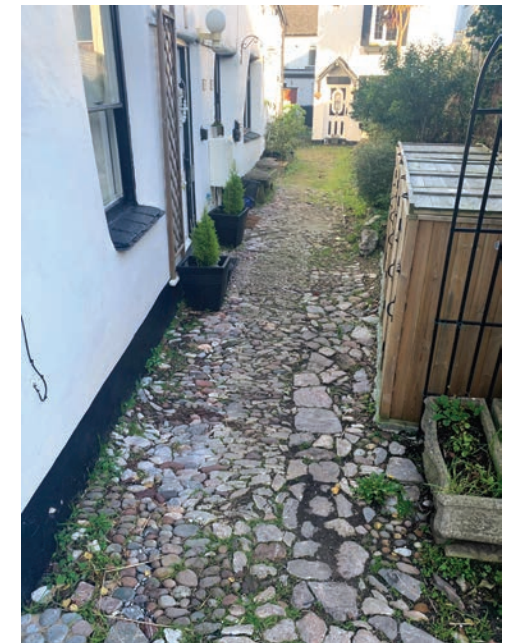
The historic cobblestones in place outside of Eaton Place.
