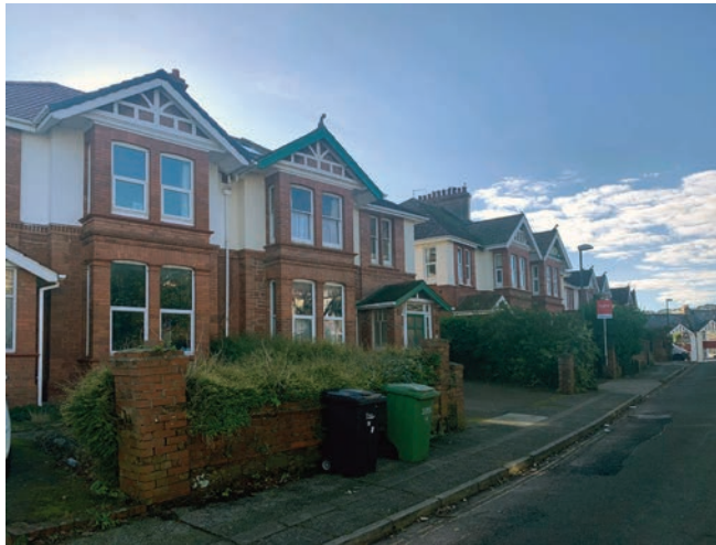
Red brick semi-detached housing on Elmsleigh Park with bay windows, rendered first floors and pitched porches.
