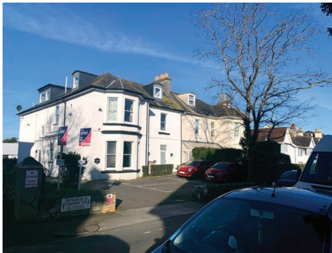
Semi-detached houses on Grosvenor Road with symmetrical canted bay windows.
