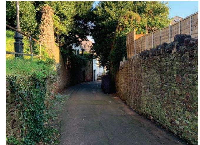
Historic red Breccia sandstone rubble boundary walls with likely medieval origins on Kirkham Street.
