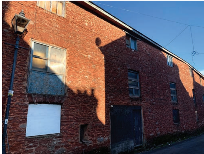
A former listed warehouse on Kirkham Street, later used as a mechanics garage and now unoccupied.
