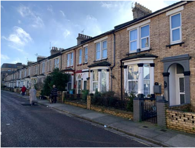
The exposed yellow brick terraces on Gerston Road. The entire street is lined on either side with houses in matching style and scale.
