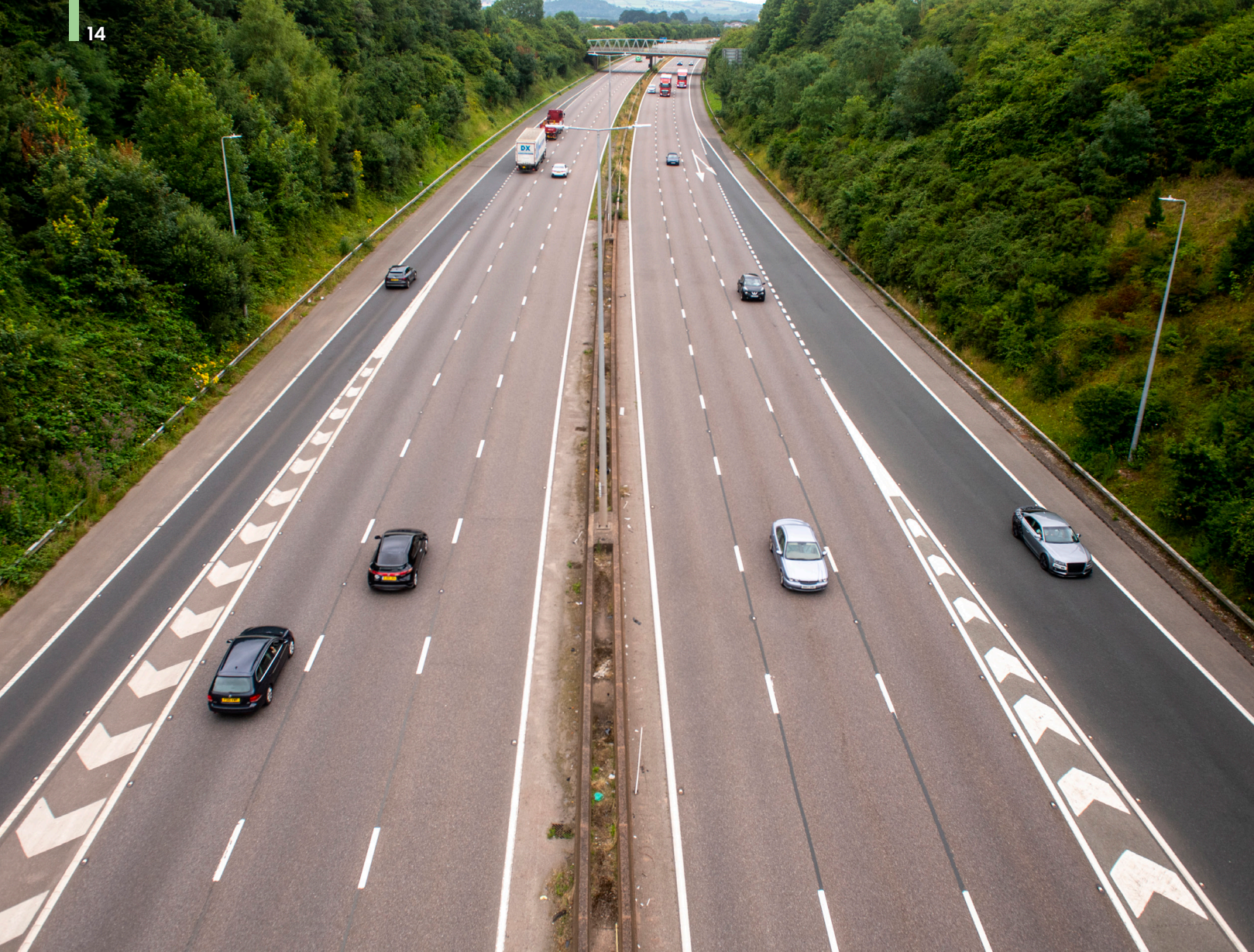
Figure 8 – Looking north from Redhayes Bridge at M5 junction 29.
