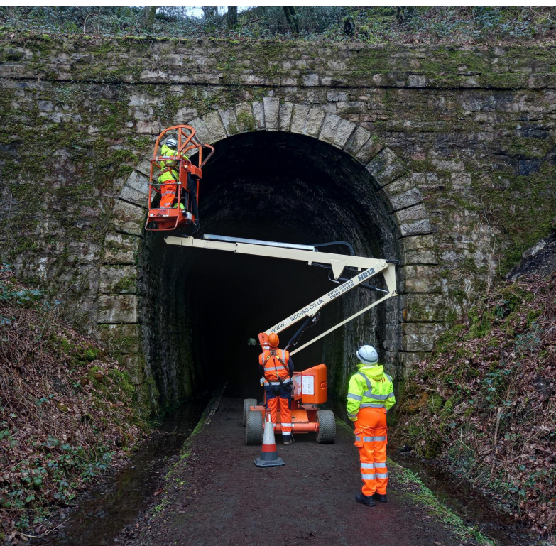
Figure 31 – Inspecting Grenofen Tunnel.
