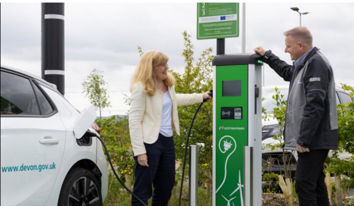
Figure 25 – Devon’s EV charging infrastructure.
