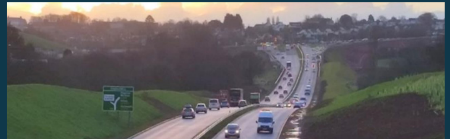
Figure 21 – South Devon Highway.
