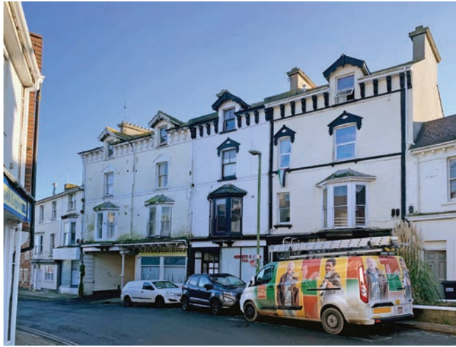
The former Crown and Anchor pub on Church Street which has been left unoccupied and been left in a poor condition.
