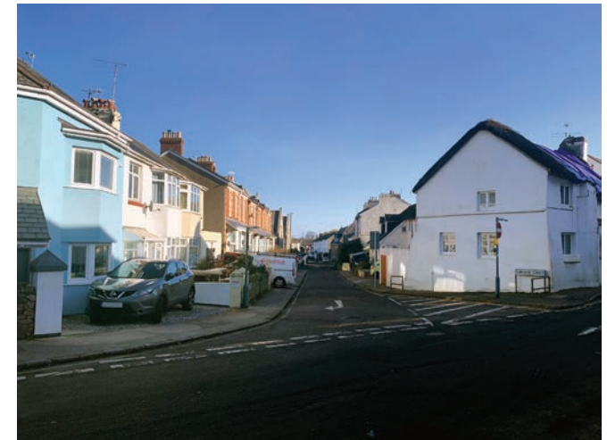
The view of Curledge Street from Fisher Street, demonstrating the variety of residential styles within the southern inner suburb of the Paignton Conservation Area.
