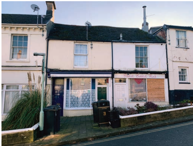
A pair of buildings on Church Street which have had their traditional shopfronts incrementally replaced with uPVC units, including the replacement of an upper floor window.
