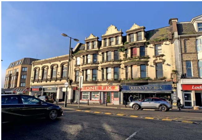
The former Bailey's Hotel on Station Square which is in a poor state of repair on the upper floors. Inoccupation has led to vegetation being allowed to grow on the front façade, windows become missing, and rainwater goods left to fail causing the building to be in a derelict condition.
