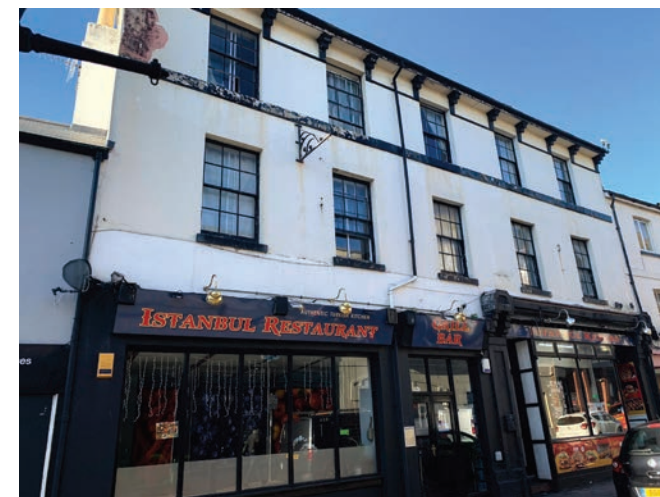
A historic shop on Winner Street which has deteriorating fabric on the upper floors, including areas of failed render and rotting timberwork including windows.
