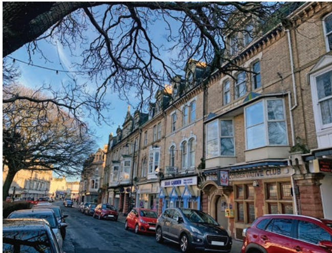
A terrace on the south side of Palace Avenue, with shops and commercial units to the ground floor and residential housing on the upper floors.
