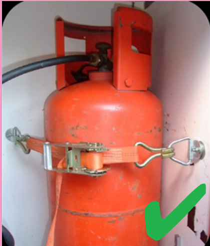
Cylinders should be secured to prevent movement during transit.
