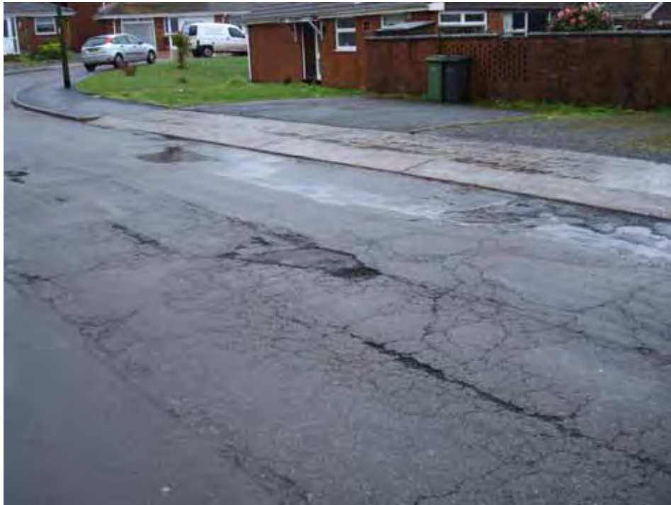
A good example of a failing carriageway in the Hookhills area. Probably created by its extensive usage by public service vehicles.
