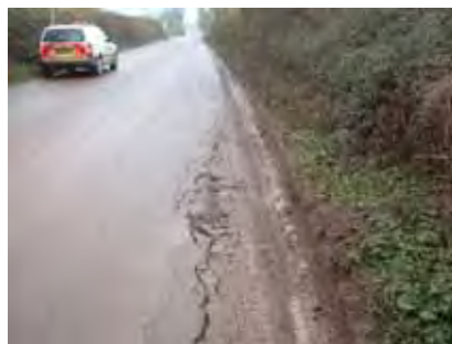
A highway inspector's van parked in the vicinity of a typical defect during a routine inspection visit.
