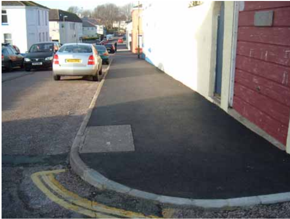
An example of a recently resurfaced footway in the Plainmoor area
