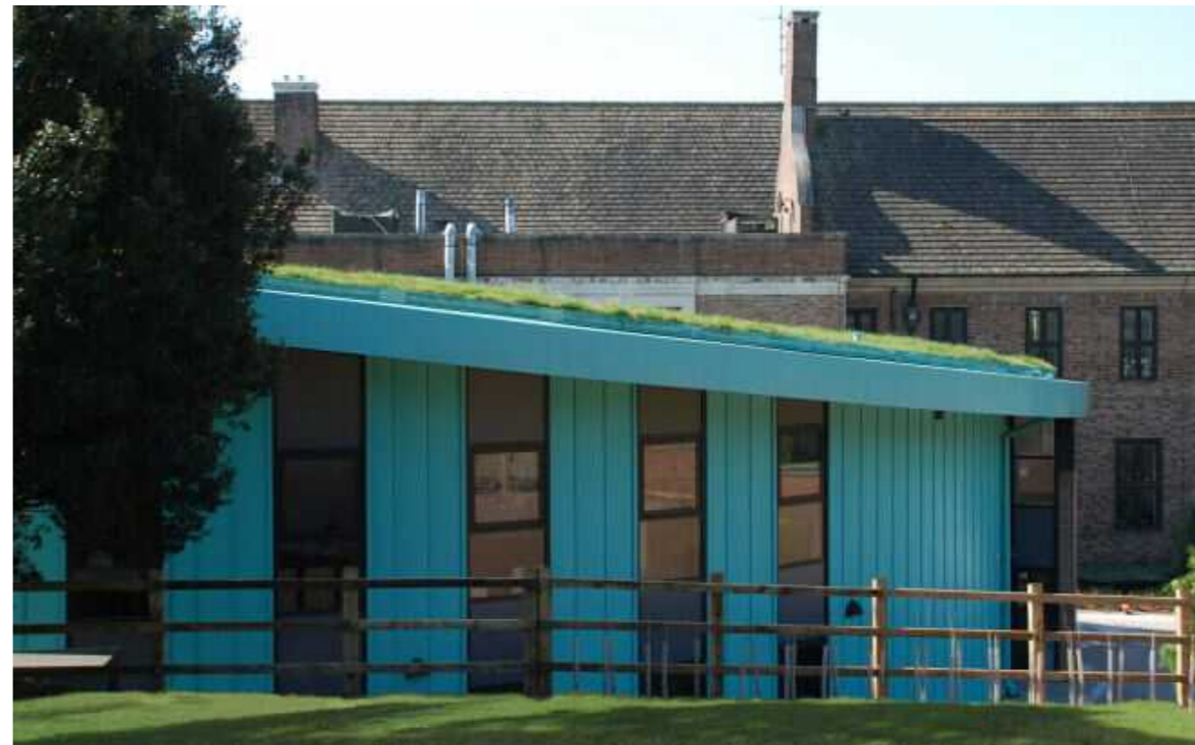
Image 3.11: An example of a successful green roof
