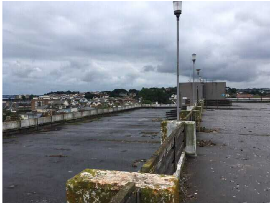
PHOTO 07: View looking south towards Queen's Park and Paignton Harbour, which can both be seen if stood at the edge of the building towards the site's southern boundary
