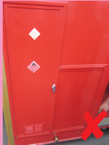
Ventilation only provided at low level. None at high level.
