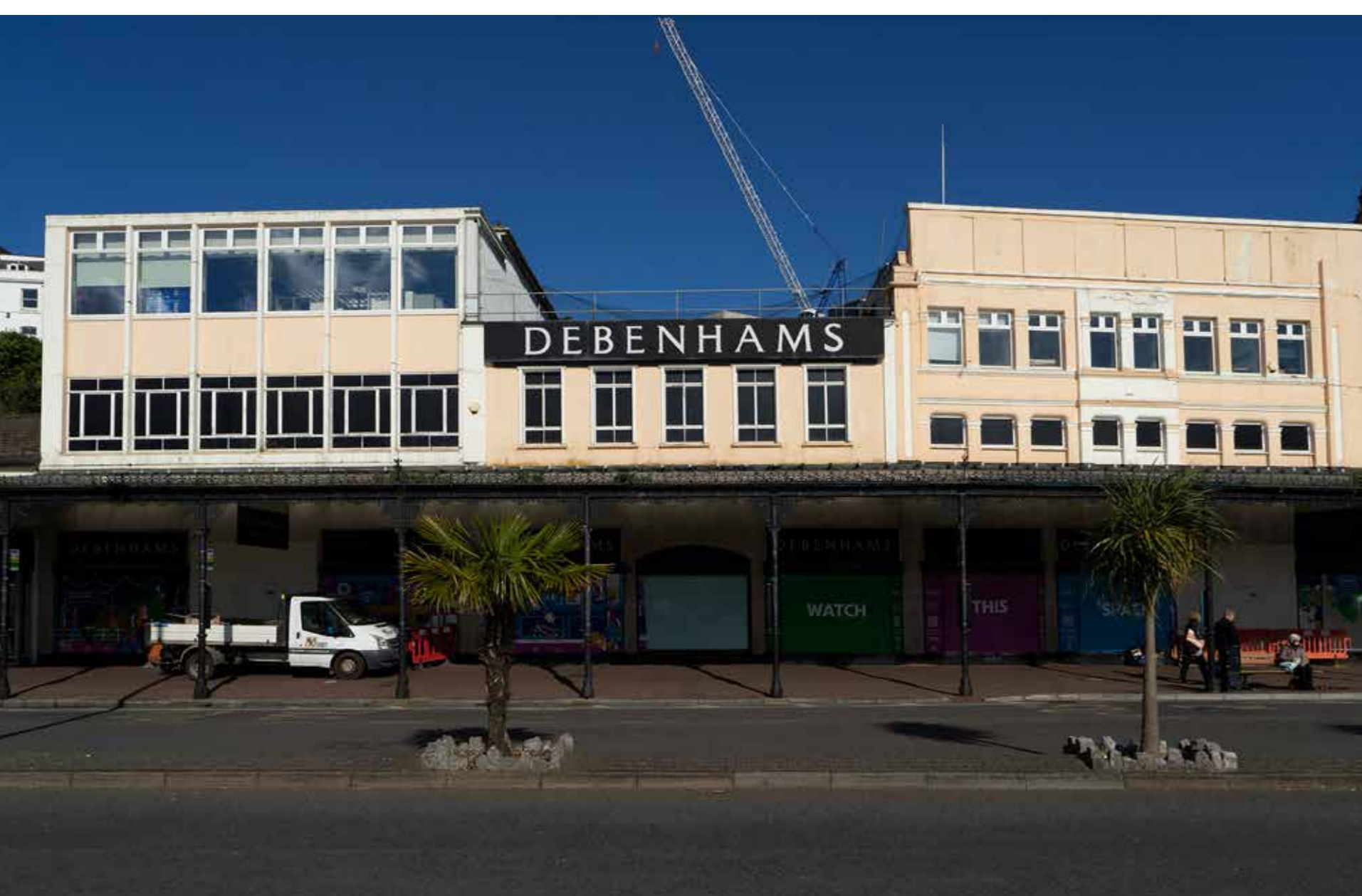
Above right: Photograph of flooding on The Strand in 2020. Image credit We Are South Devon Above: Debenhams current elevation. Image credit Sanders Studio
