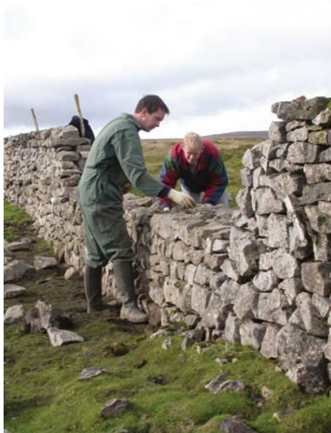
Repairing a section of drystone wall
