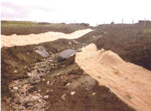
Peatland restoration work, Peak District
