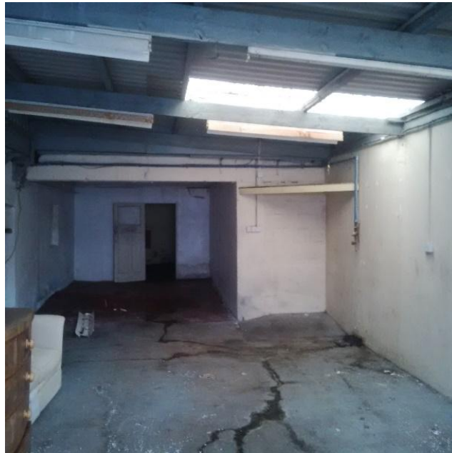
Figure 7 - Old Dairy, interior of former office space 2
