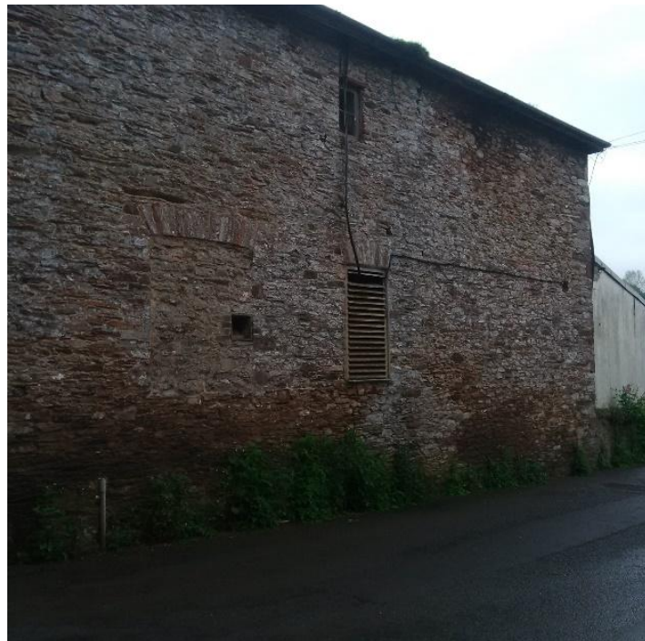
Figure 4 - Old Dairy, view from north
