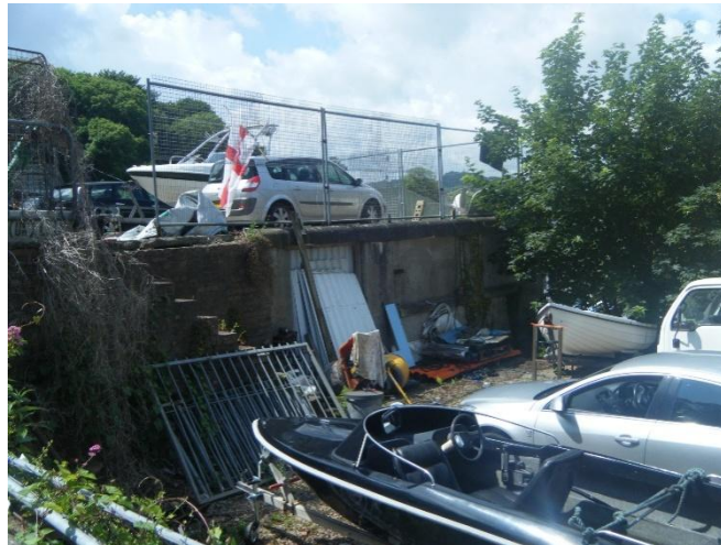
Figure 15 Paint Factory – surveyed structure, view from west
