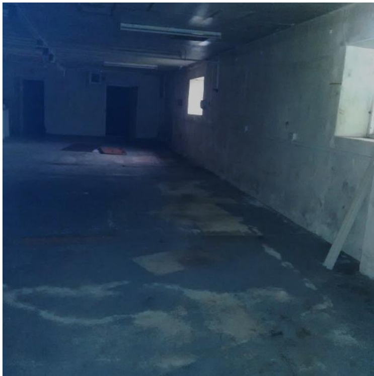
Figure 6 - Old Dairy, interior of former office space 1
