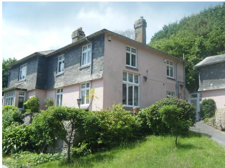
Figure 17 - Kings Barton, view from north-east
