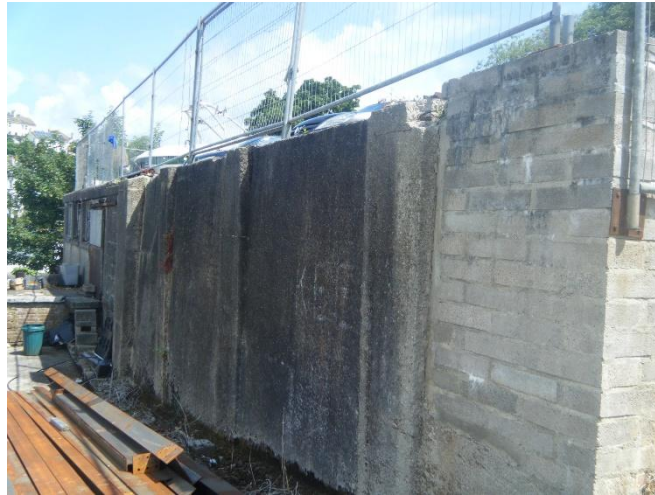
Figure 14 Paint Factory – surveyed structure, view from north-west
