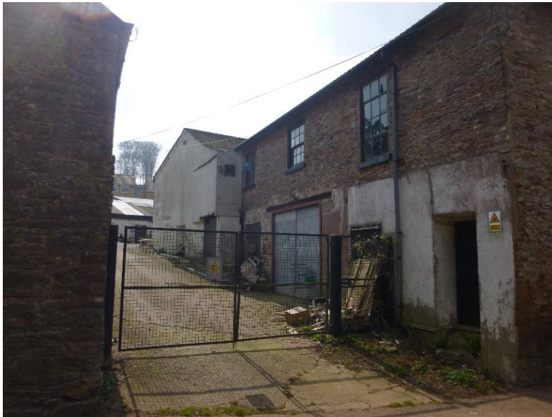
Figure 5 - Old Dairy, view from north-east
