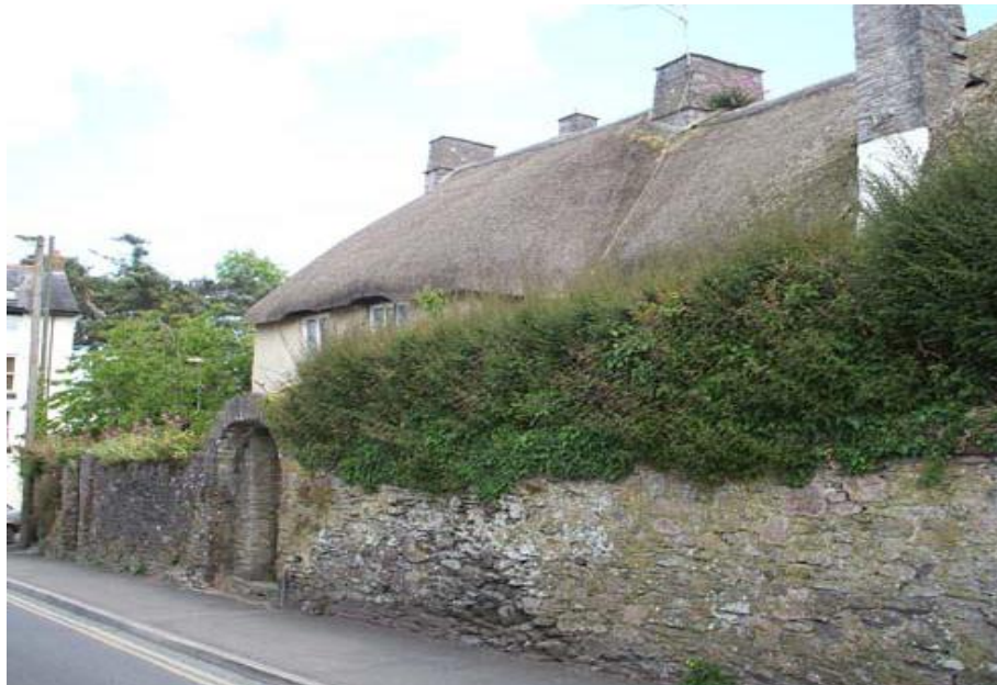
Figure 41: Hearthstone is a large through-passage early post-medieval thatched house now sub-divided. High hedges and trees above high walls enclose the lower house from public view. Wall, arch and chimney are all in local stone; the walls are in cob and stone.
