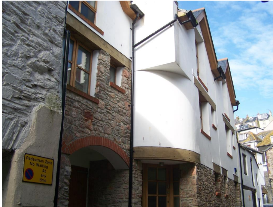
Figure 16: A sympathetic well-designed example of a Mews development in Pump Street off Fore Street.
