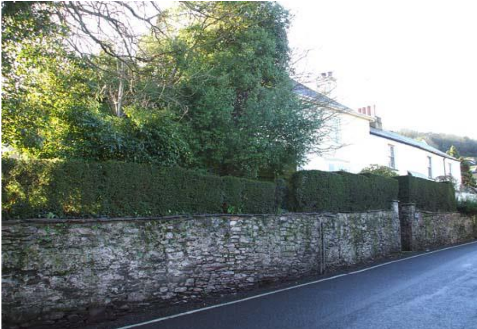
Figure 32: Upper Milton Street, showing the high Devonian limestone walls — rubble-built walls are typical of much of this part of Brixham where they act as boundaries and terraces; the mature hedges above add to the sense of enclosure.
