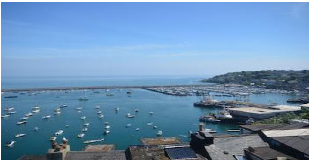
Figure 23: Roof top view from Furzeham over Brixham outer harbour with the Marina and Breakwater in the background.
