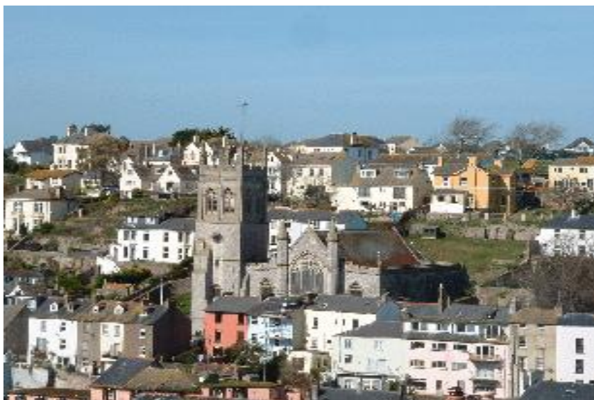
Figure 6: All Saints Church Brixham showing the variety of houses surrounding it.
