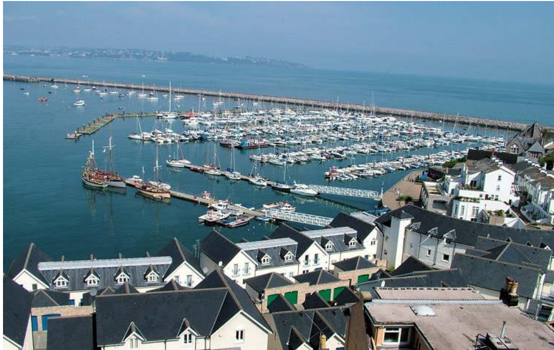
Figure 9: Brixham Marina with Moorings Reach development and the heritage pontoon in the foreground and Brixham Breakwater in the background.
