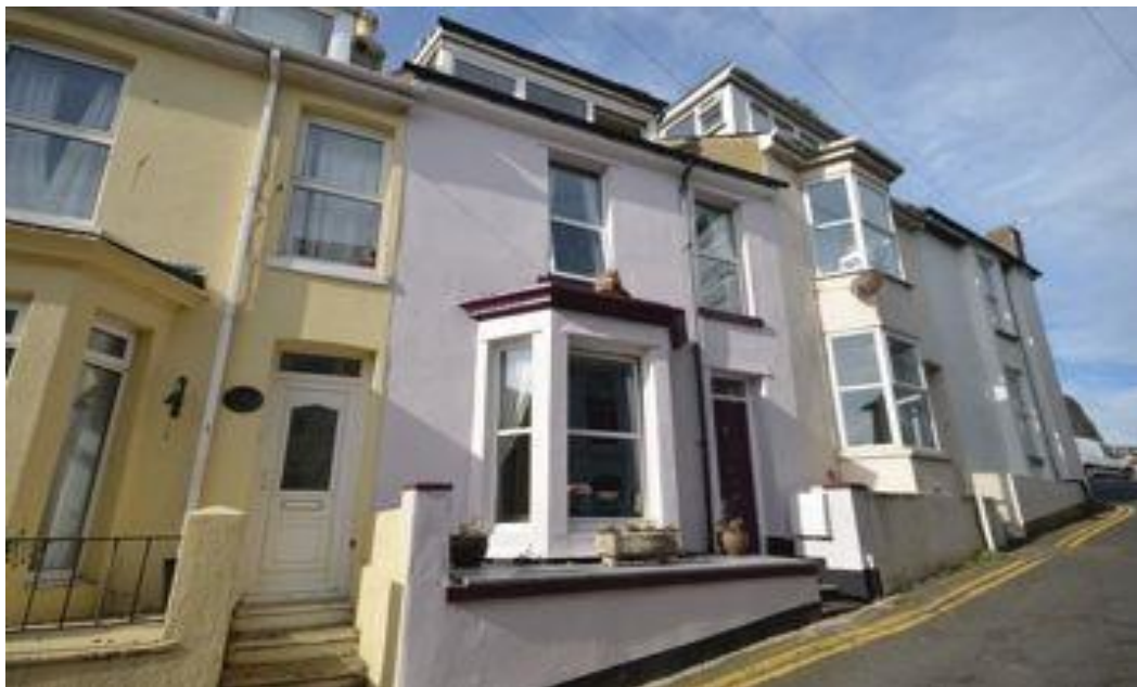
Figure 26: Typical style of terraced housing in North Furzeham Road showing roof-top dormer extensions.
