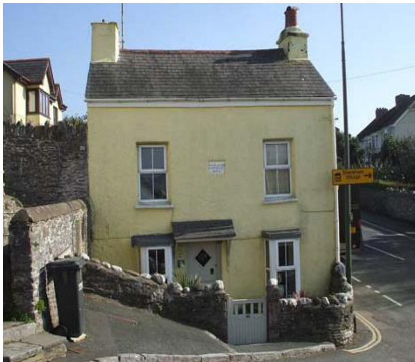
Figure 37: Roseacre Cottage dated 1836 half-terraced into the hill.
