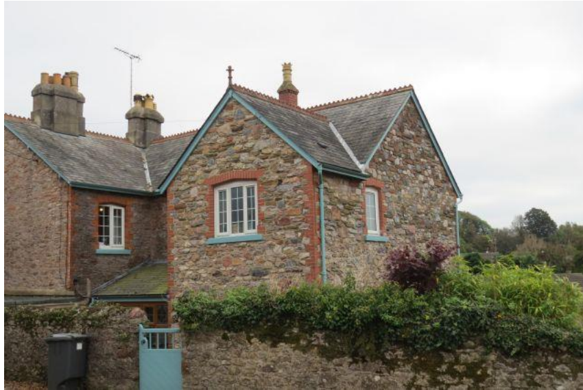
Figure 41: Good example of recent extension which sensitively accords with the existing style and materials of this Victorian house in the Stoke Gabriel Road.
