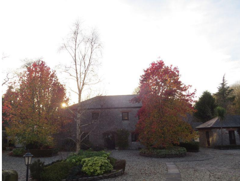
Figure 43: Positive example of attractively landscaped barn conversions at Manor Farm, AONB, using and adapting original materials and design.
