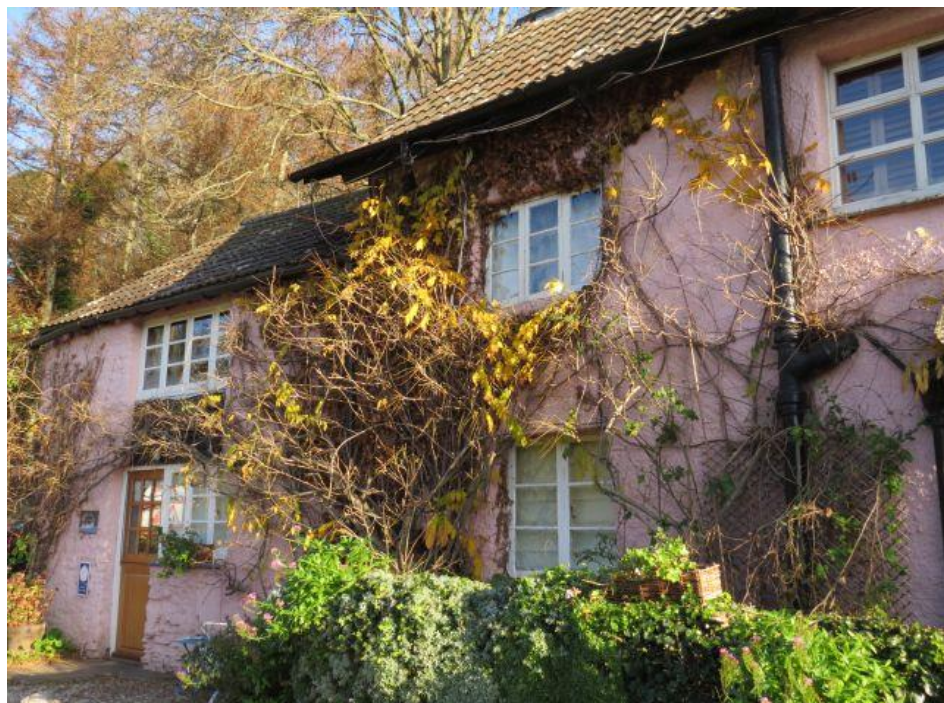
Figure 20: Port Hill Cottage, Stoke Gabriel Road, 17th century vintage, with rare stone spiral staircase.
