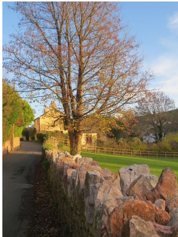
Figure 42: Respectful restoration of limestone wall at the AONB end of Stoke Gabriel Road, which replicates the regionally authentic "cock and hen" structure.
