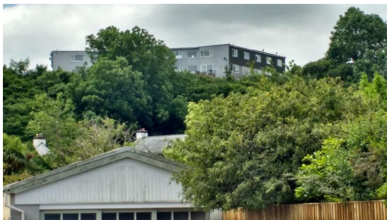
Figure 19: Skyline from Broadsands Avenue with overmassed building.
