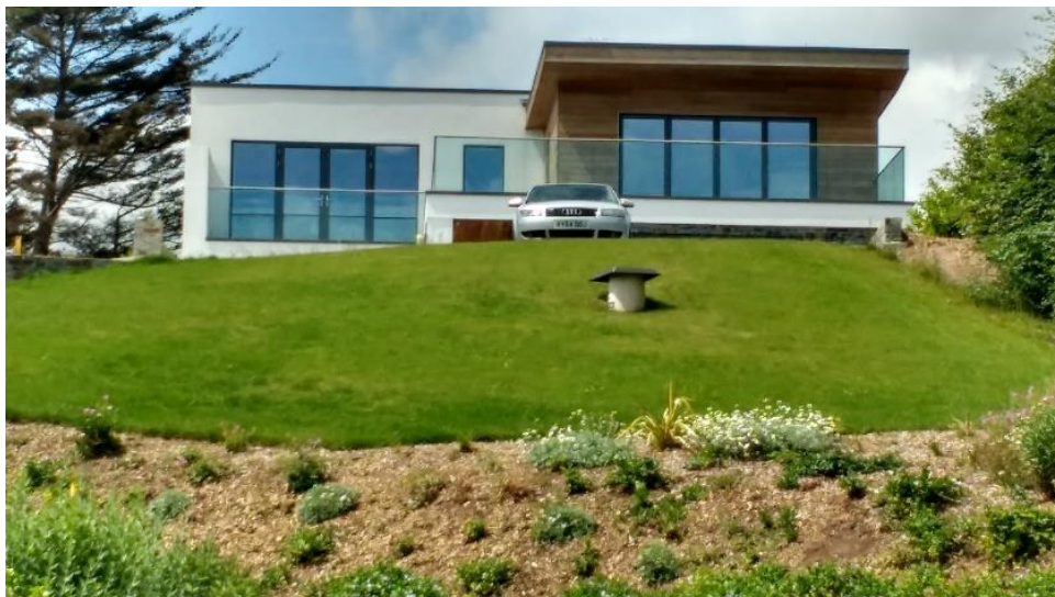
Figure 24: Appropriate high design standard in the new construction at Waterside.
