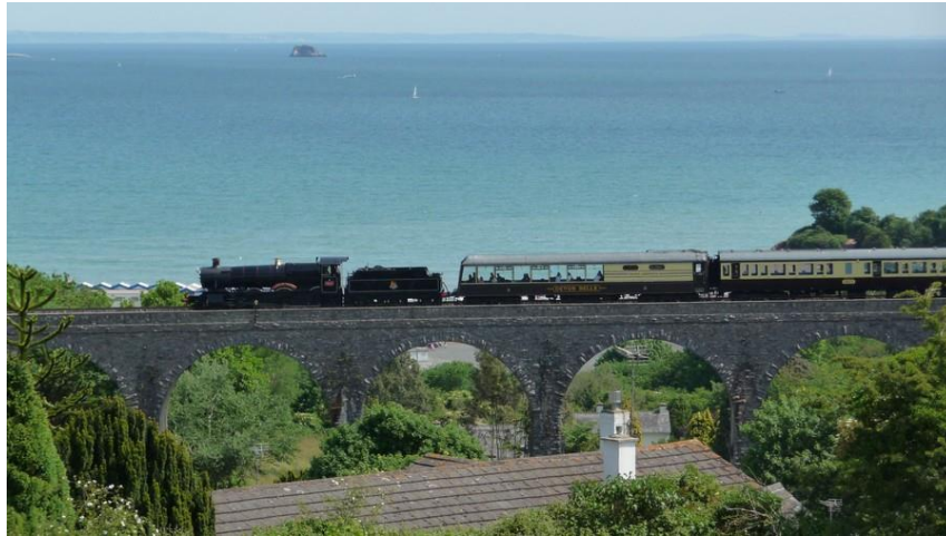
Figure 3: Brunel viaduct at Broadsands.
