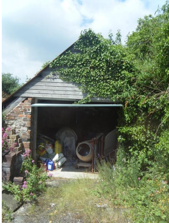
Figure 10 - Knapman's Yard, building 2
