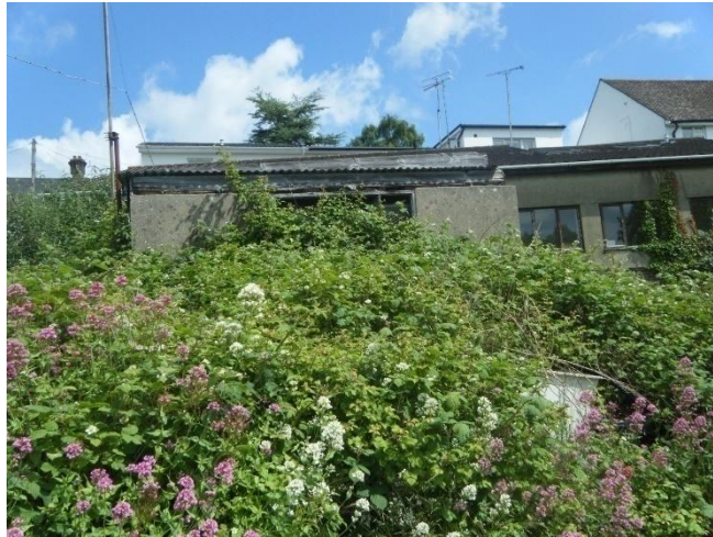
Figure 12 - Knapman's Yard, building 5
