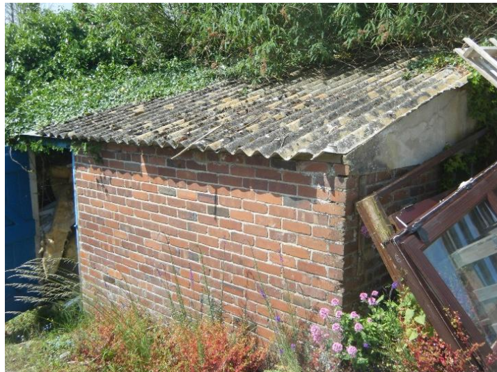
Figure 9 Knapman's Yard, building 1
