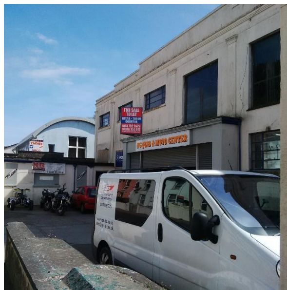
Figure 10 The former Jewson Builders' Merchants
