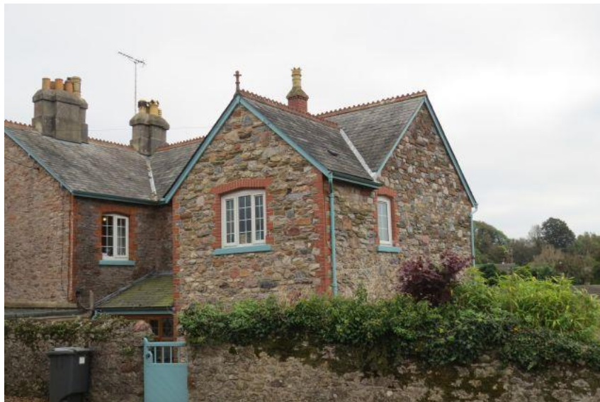
Figure 41: Good example of recent extension which sensitively accords with the existing style and materials of this Victorian house in the Stoke Gabriel Road.
