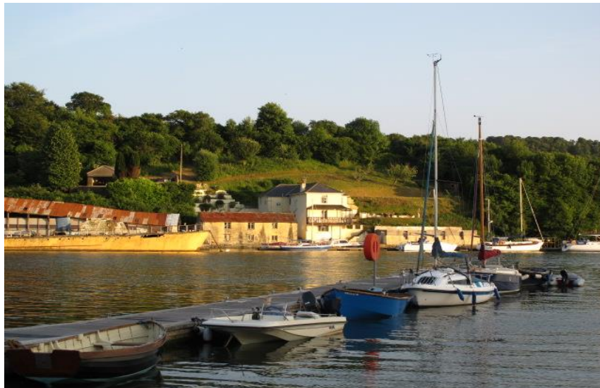
Figure 2: Galmpton Creek, showing Dolphin Quay with marine units and additional pontoon for leisure craft.
