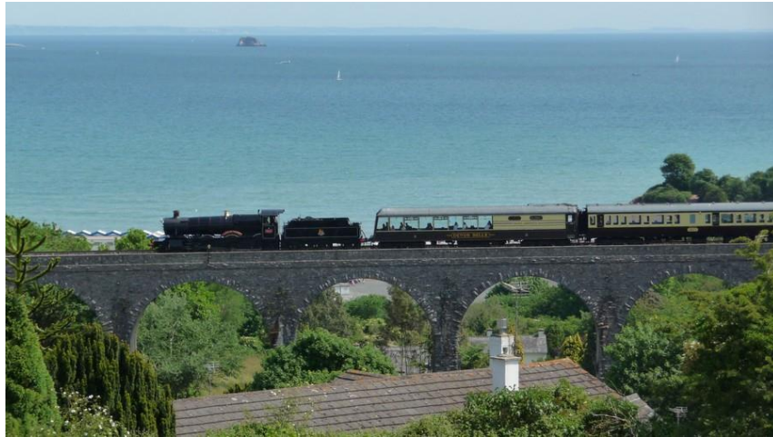
Figure 3: Brunel viaduct at Broadsands.
