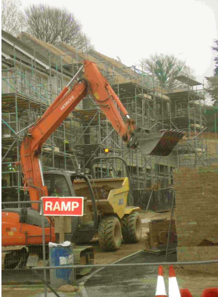
Housing under construction in 2007, Paignton
