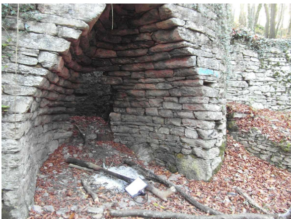
Photo 5 – one of the two lime kilns in The Grove
