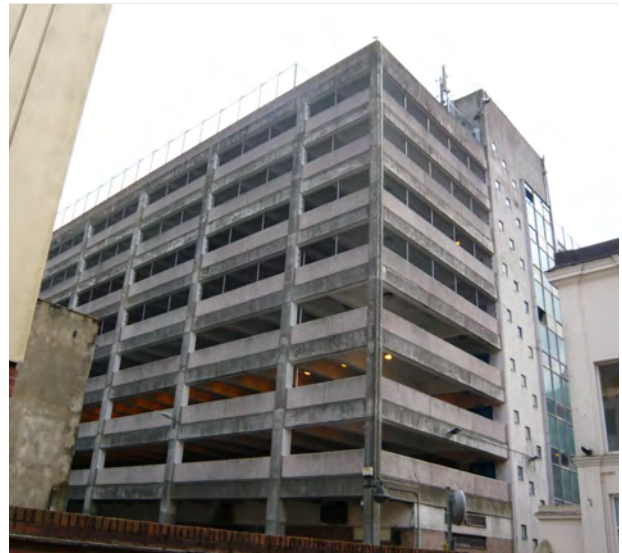
Union Street Car Park is an important opportunity site
