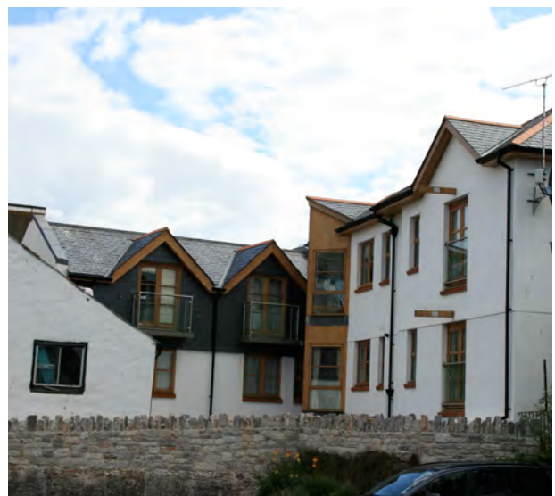
Sympathetic town centre infill development
