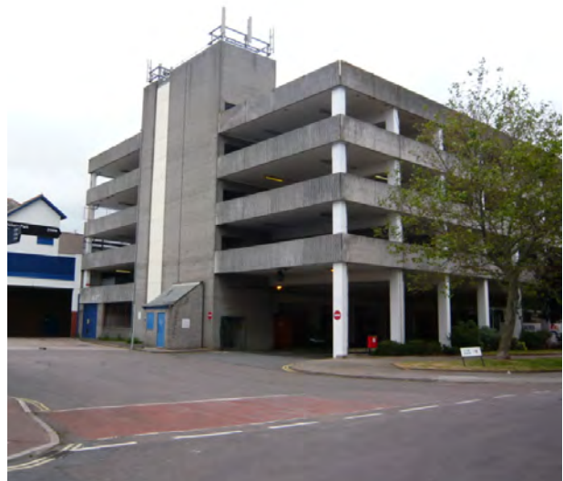
Car Park as part of Victoria Shopping Centre site
