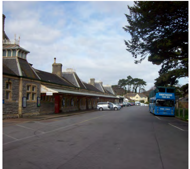
Single storey building at Torquay Station
