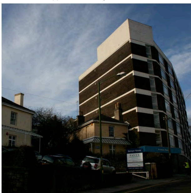
Roebuck House is tall compared to its 2 storey neighbours
