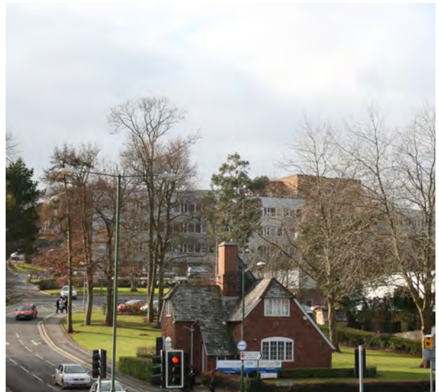
Torbay Hospital is a tall, large building in a prominent location on a hilltop
