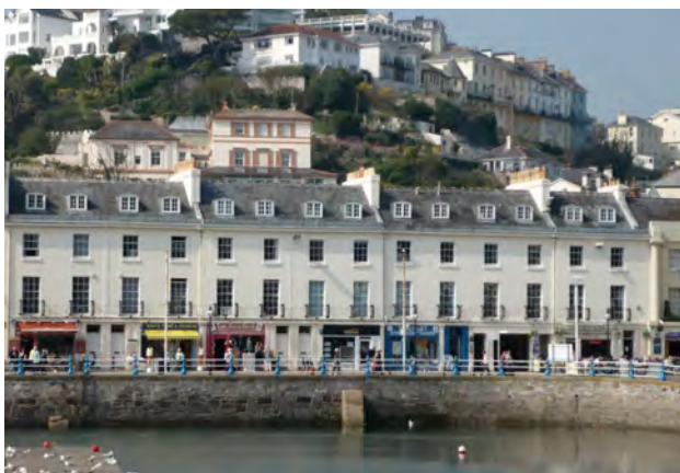
The Coastal Zone is typified by 3 storey buildings, often with roofspace accommodation
