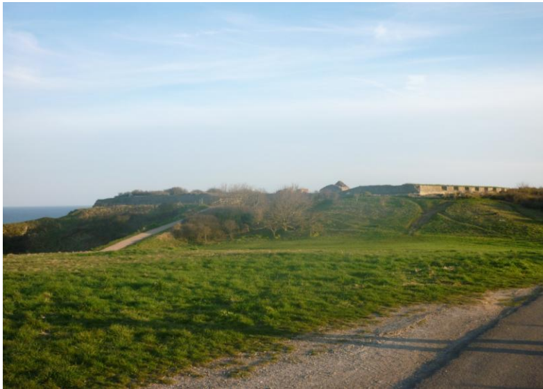
View looking south towards Fort no 1
