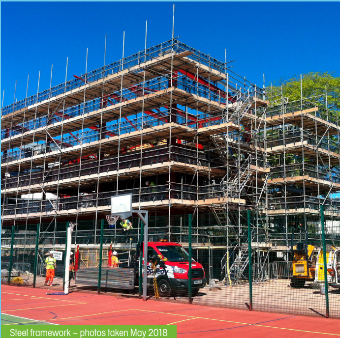
Steel framework – photos taken May 2018
