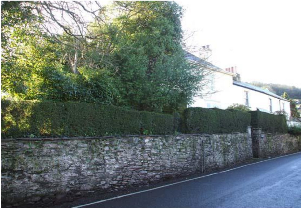
Figure 32: Upper Milton Street, showing the high Devonian limestone walls — rubble-built walls are typical of much of this part of Brixham where they act as boundaries and terraces; the mature hedges above add to the sense of enclosure.
