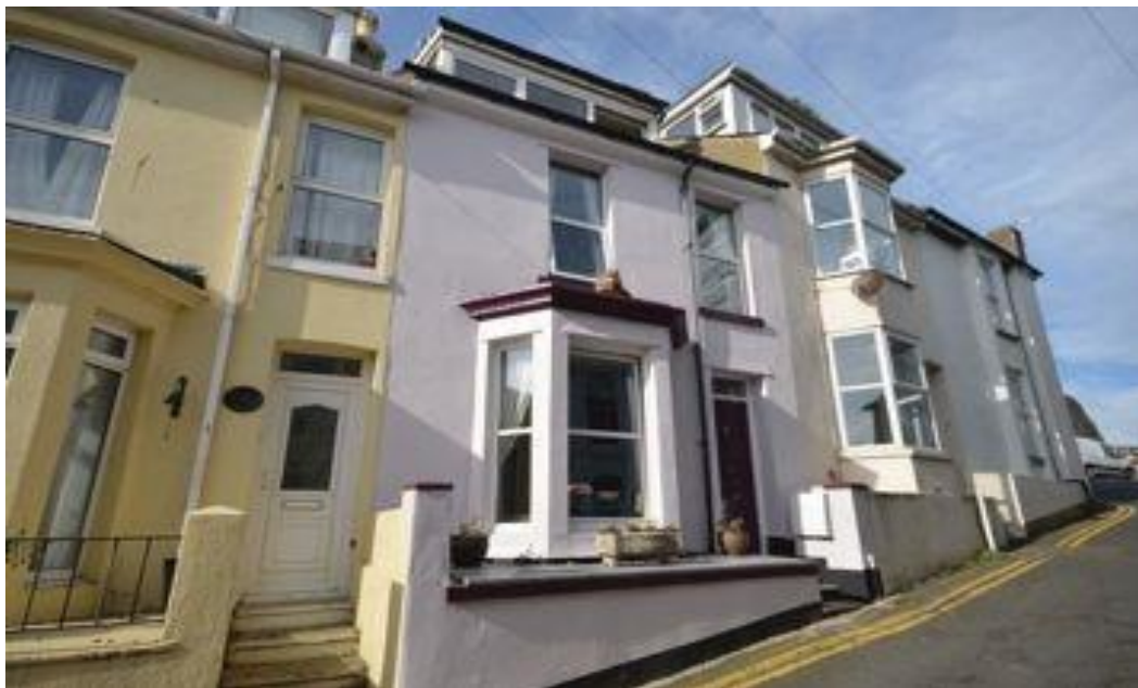
Figure 26: Typical style of terraced housing in North Furzeham Road showing roof-top dormer extensions.
