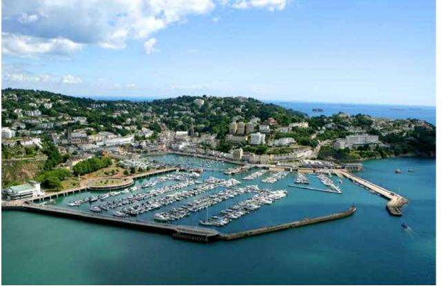
of its seaward face as well as raising the breakwater's height by 50cm is expected to substantially improve its utility as a breakwater and future-proof it against rises in sea level due to climate change for up to 50 years.
