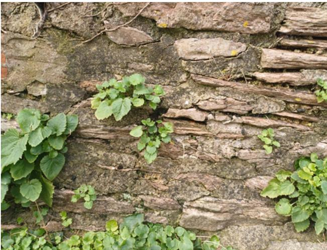
Detail of a boundary which has been repointed with non-breathable cementitious mortar and has extensive vegetation growth. A plant will typically root in mortar joints and force itself deeper as it grows, which can push the built fabric out of position and weaken the integrity of the wall.
