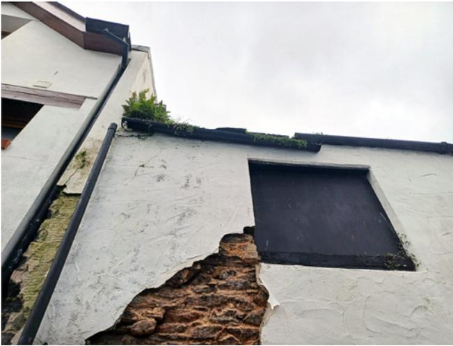
An example of a blocked and broken gutter and failing render to a property on Pump Street.
