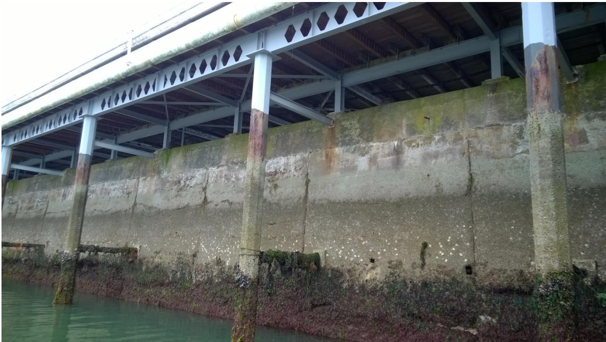
2 1970s-installed galvanised steel frame below timber boardwalk supported on the original concrete and masonry pier, and by steel piles (columns)
