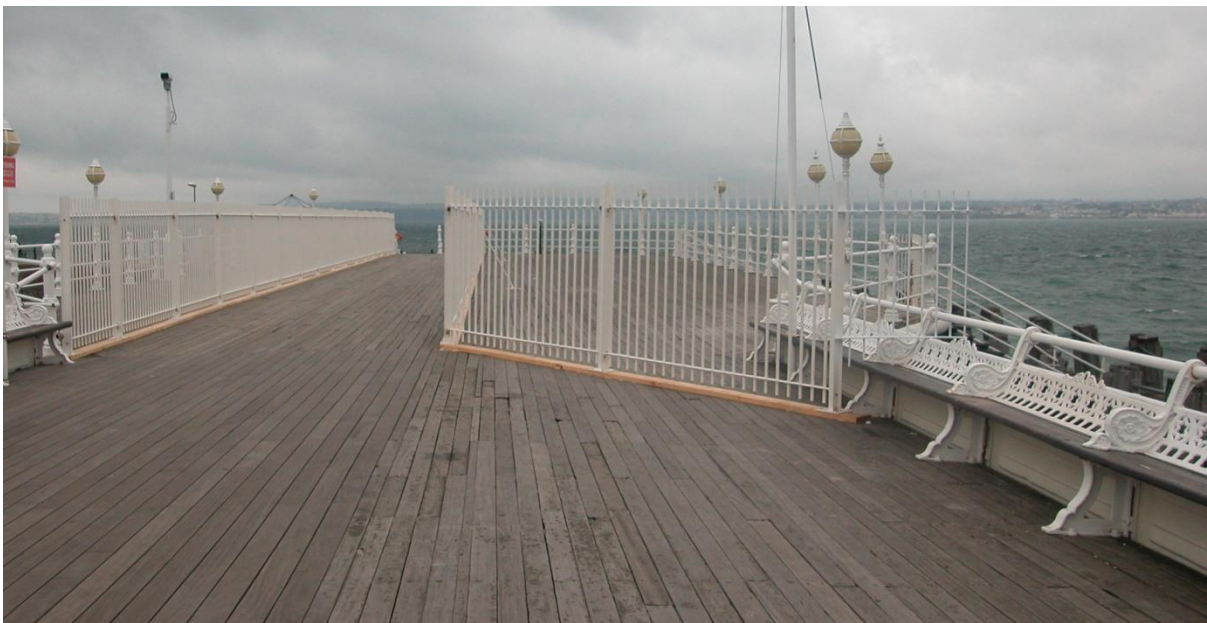
3 Widening at the pier head; fencing installed in 2007 to close unsafe areas, thoroughfare maintained for public access to pier beyond
