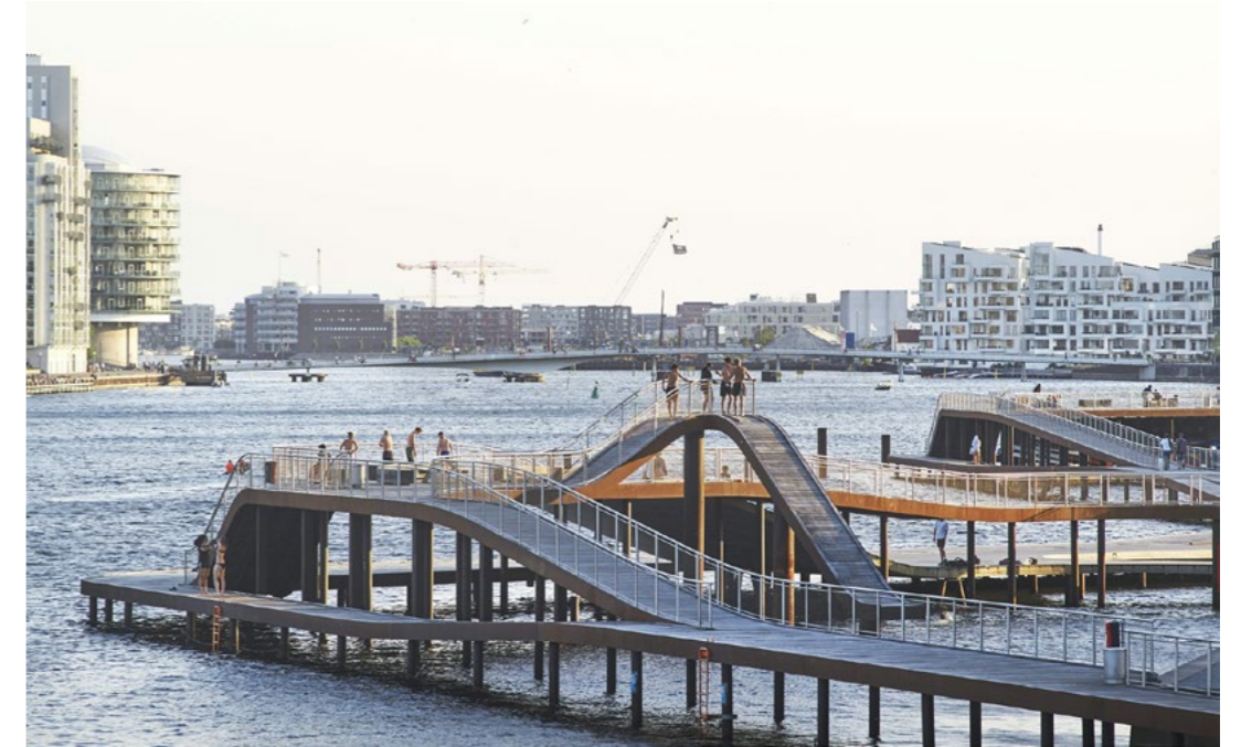
Kalvebod, Copenhagen, boardwalk
