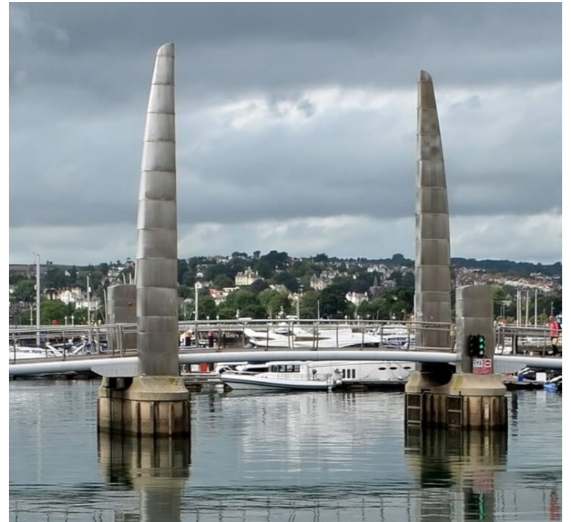
Torquay Marina Bridge
