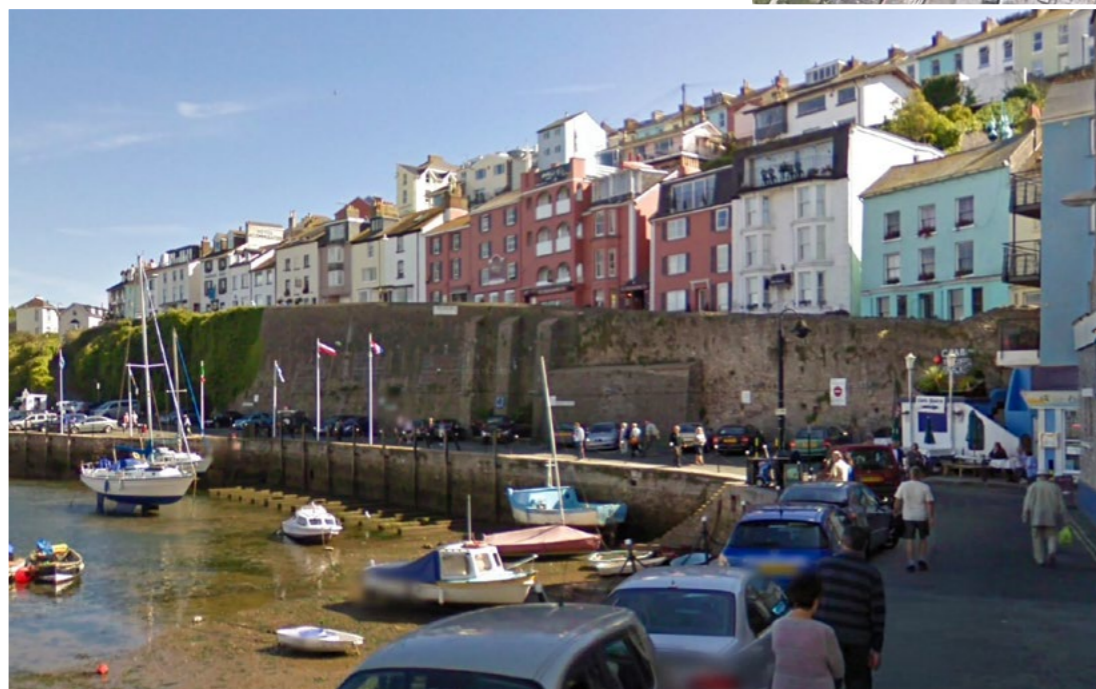
South Quay, the blank retaining wall - a blank canvas opportunity.
